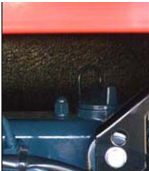
Image 2-10 Oil level check
